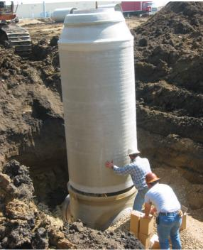
Introducing a new Adhesive Joint for fiberglass manholes and wetwells with a concrete slab base. Fiberglass manholes and wetwells require the use of a concrete base to offset buoyancy. This innovative joint allows CSI to deliver manholes or wetwells with concrete slabs to a site ready for installation. The barrel is connected on-site to the base at the adhesive channel. Installation times can be reduced by more than 60% in some cases.
