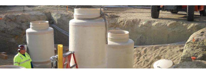
Underground petroleum storage tanks are not getting any smaller and as capacity grows, so does the need for larger tank sumps. To meet market demand, Containment Solutions offers a 54" double-wall tank sump. The spacious interior eliminates the need for a second tank sump in dual submersible or high capacity pump applications. Fitting two pumps on one tank manway saves significant time and money.
