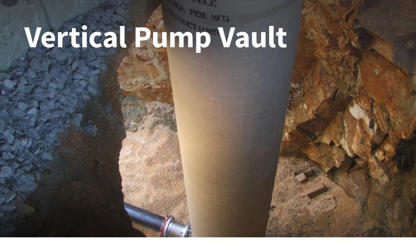
Containment Solutions™ vertical pump vault and tank meets the requirements of NFPA 22 for the storage of fire protection water. The fiberglass pump vault can be installed along with a Flowtite® fiberglass tank to complete an underground fire protection storage system. This installation method allows 100% of the tank volume to be accessible.
