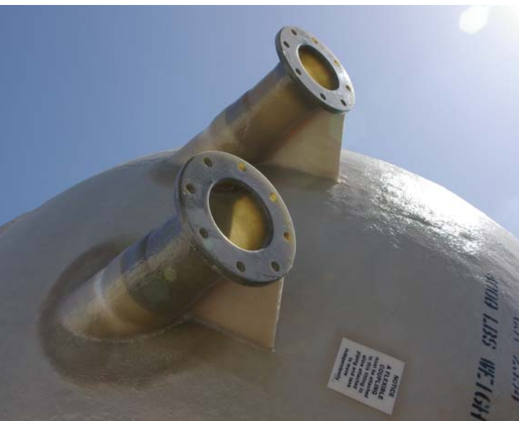
▼ FIBERGLASS NOZZLES AND PVC PIPING
