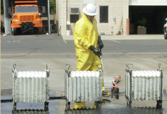
Oleophilic coalescer plate packs are intended to be removed for cleaning. The number of plate packs will vary based on tank size and required effluent quality.
