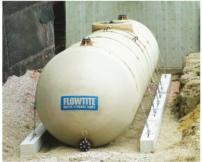
Piping connects to a flanged nozzle on the Flowtite tank to facilitate the transfer of water to the fire protection system.
