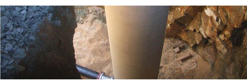
Containment Solutions' vertical pump vault and tank meets the requirements of NFPA 22 for the storage of fire protection water. The fiberglass pump vault can be installed along with a Flowtite® fiberglass tank to complete an underground fire protection storage system. This installation method allows 100% of the tank volume to be accessible.
